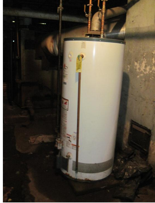
Existing DHW Heaters
