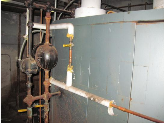
Existing Steam Boiler
