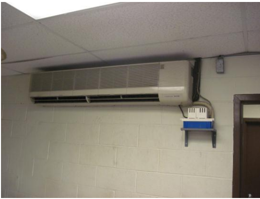
Existing Split AC Units
